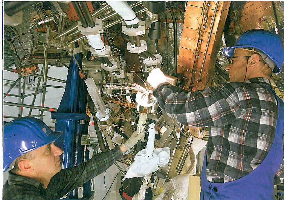
Difficult connection: specialists from Cracow (IFJ PAN) install the complex superconducting coils of Wendelstein 7-X. (Picture: IPP, Anja Richter Ullmann)
